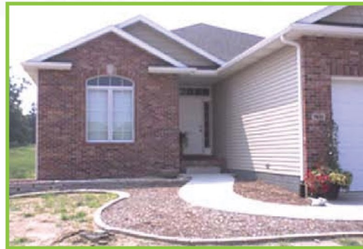
House built without LOW-E
