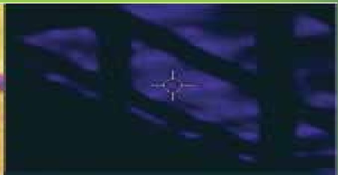
Thermal imaging of the same attic WITH ThermaSheet® roofing underlayment. Temperature is 98°
